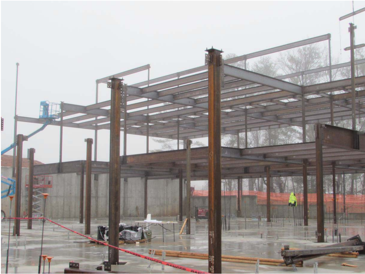
Structural Steel Lower level
