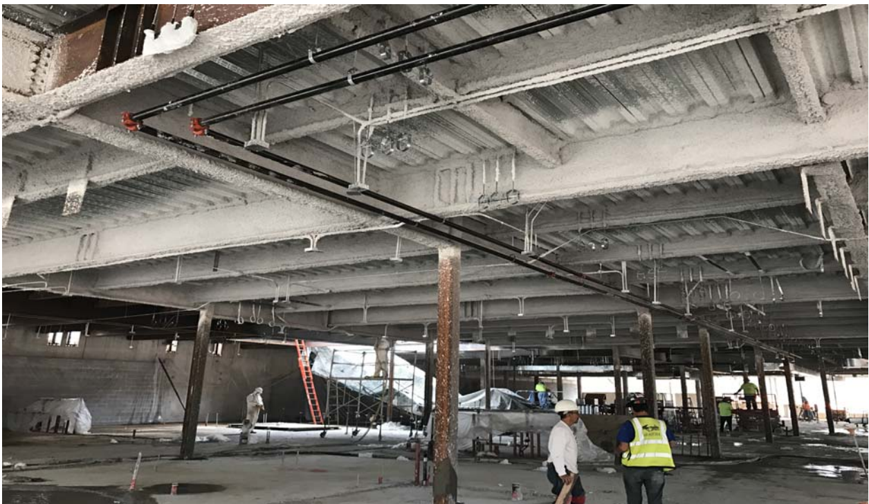
Lower Level Fireproofing
