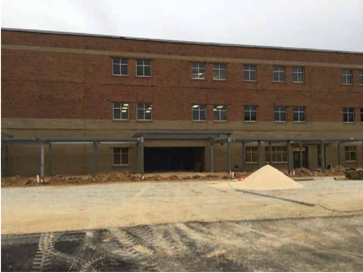
South view at rear canopy.
