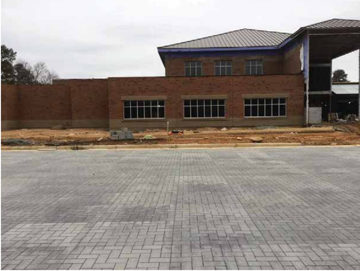
Front view at main entrance.
