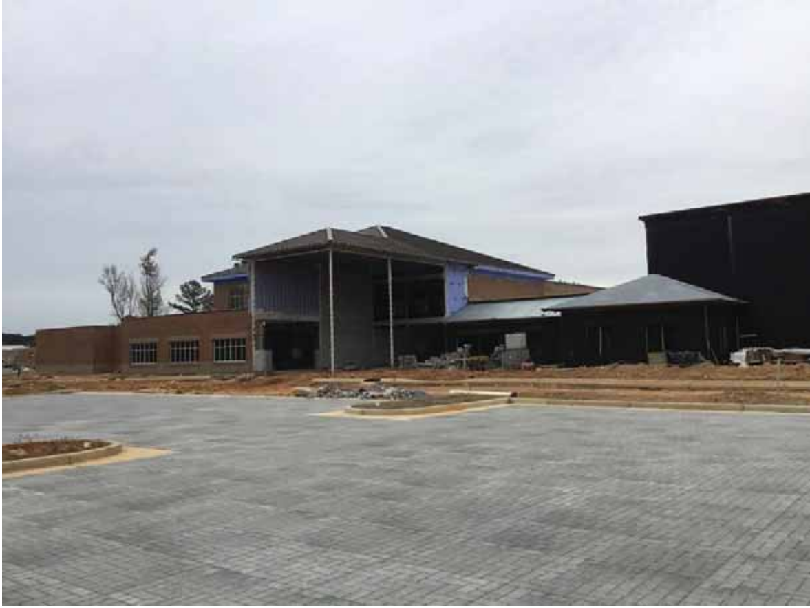
Front view at building.
