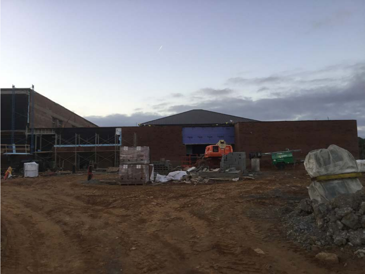
North view at main level.
