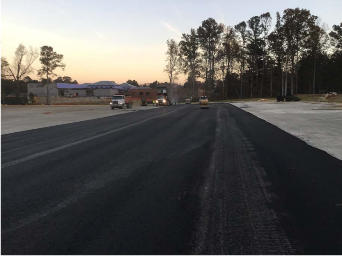
Paving process at bus parking.
