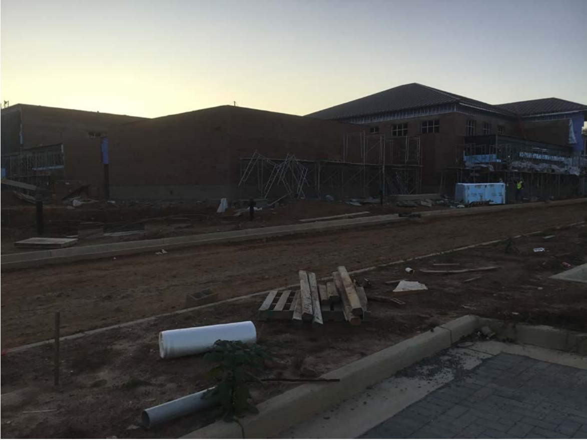
West view at North side of kitchen.
