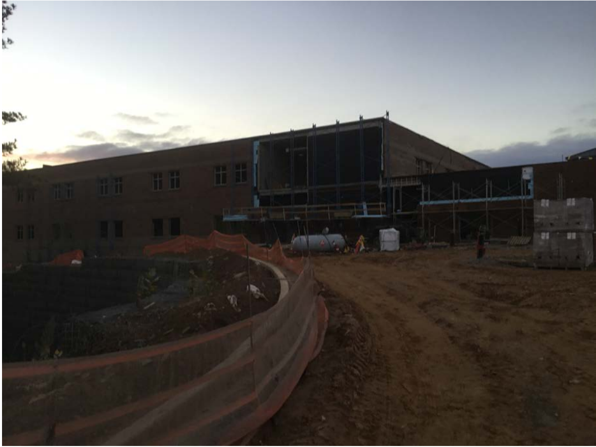
North view at 2 story.
