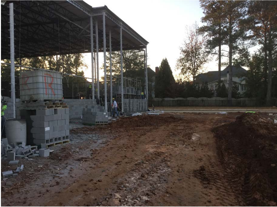
West view at auditorium.
