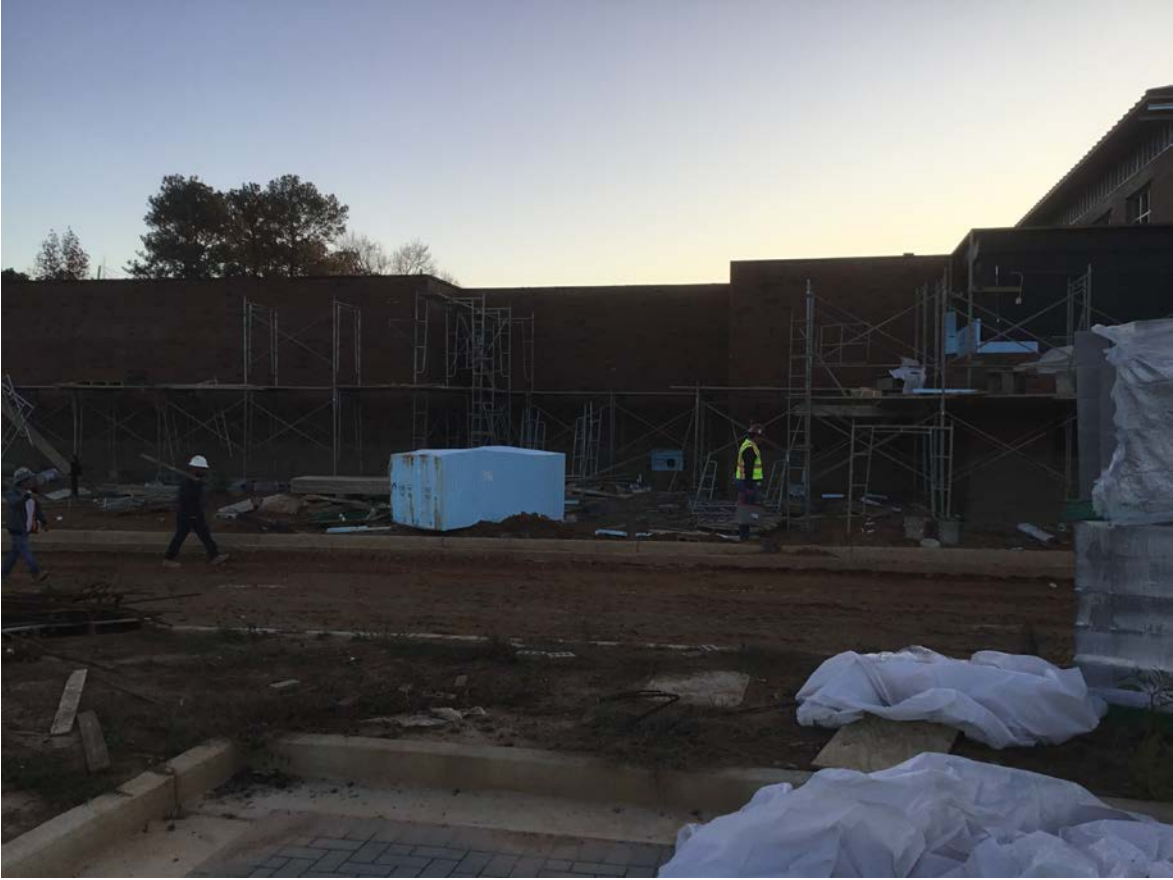
West view at kitchen area.
