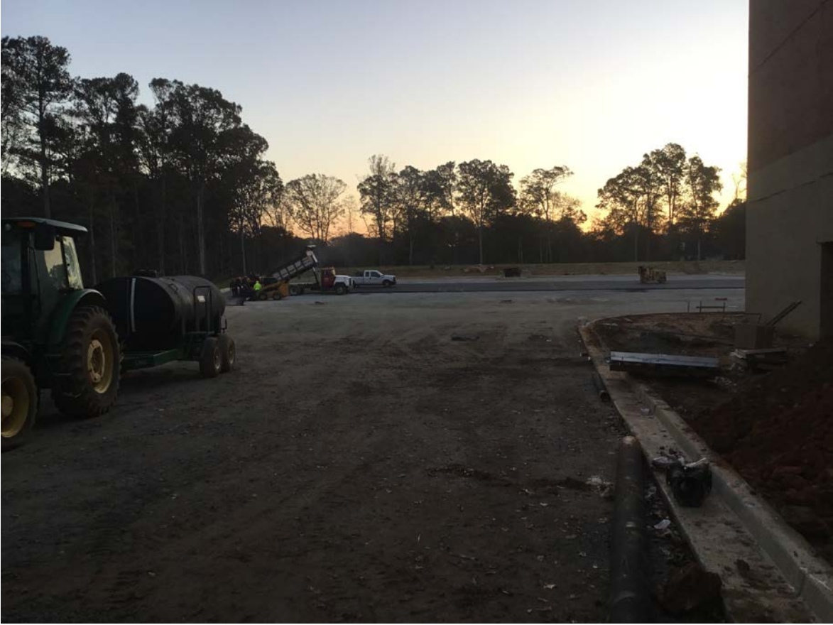
North view at 3 story facing bus parking.
