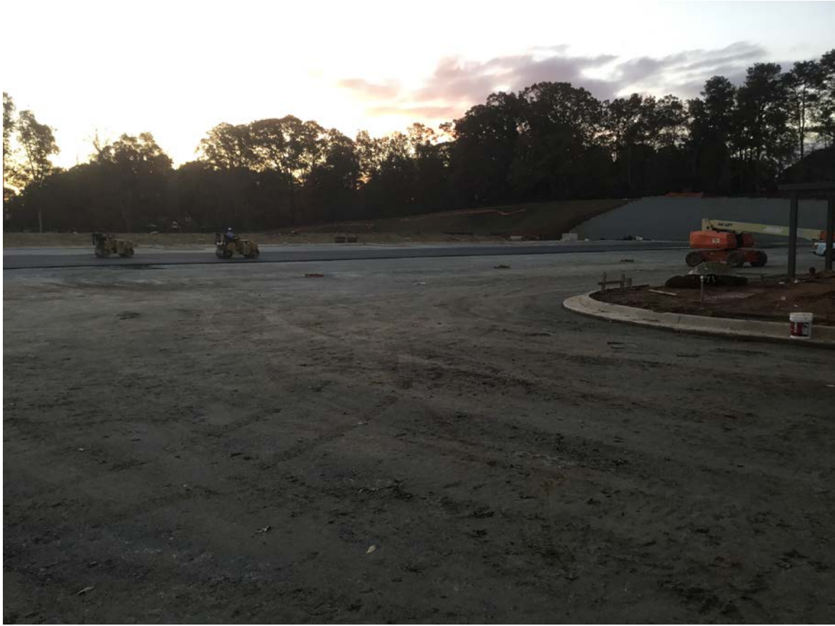
North side of bus parking facing east.
