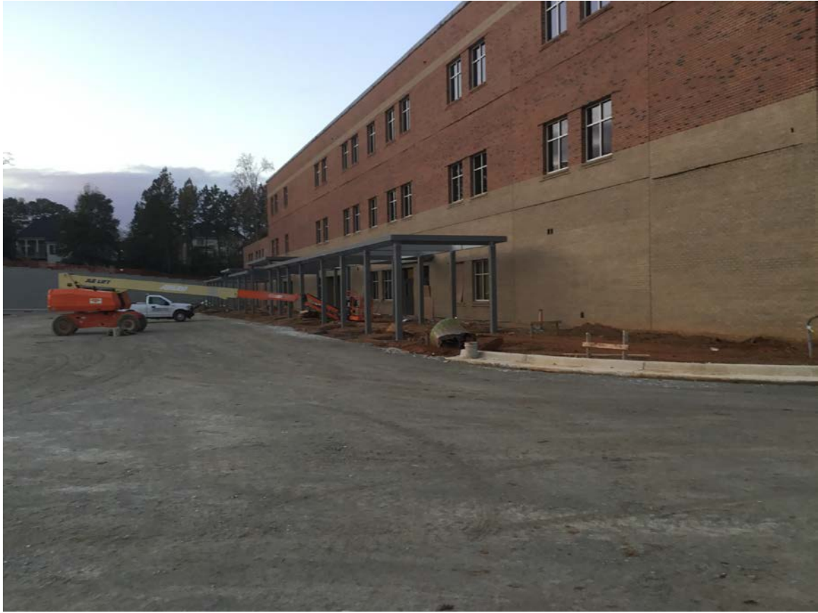
East side of 3 story facing south.
