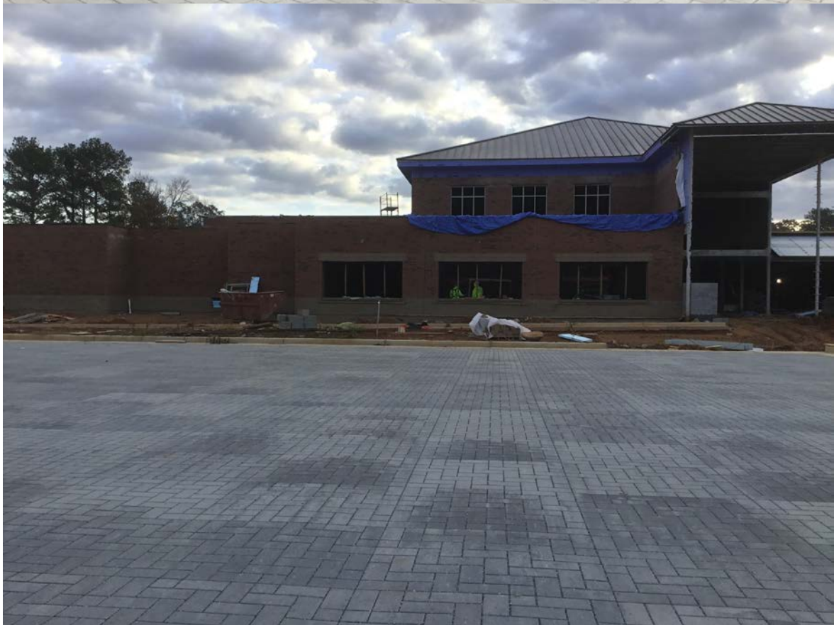
West view at main entrance
