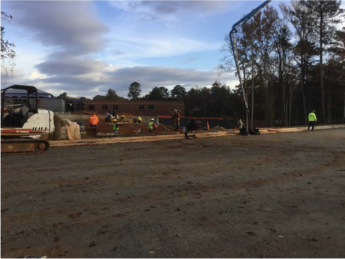
Concrete spillway being built
