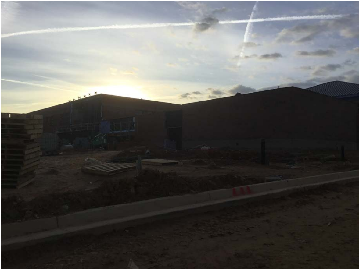
Northwest at kitchen area
