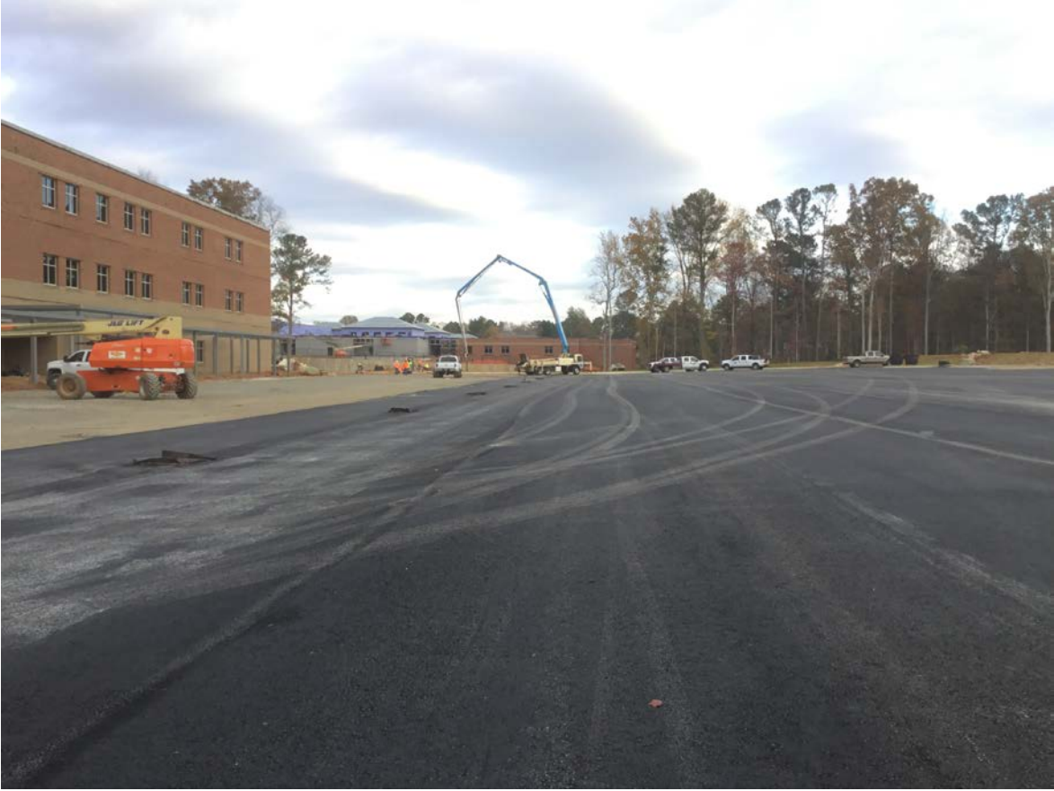
Northward view at bus parking area
