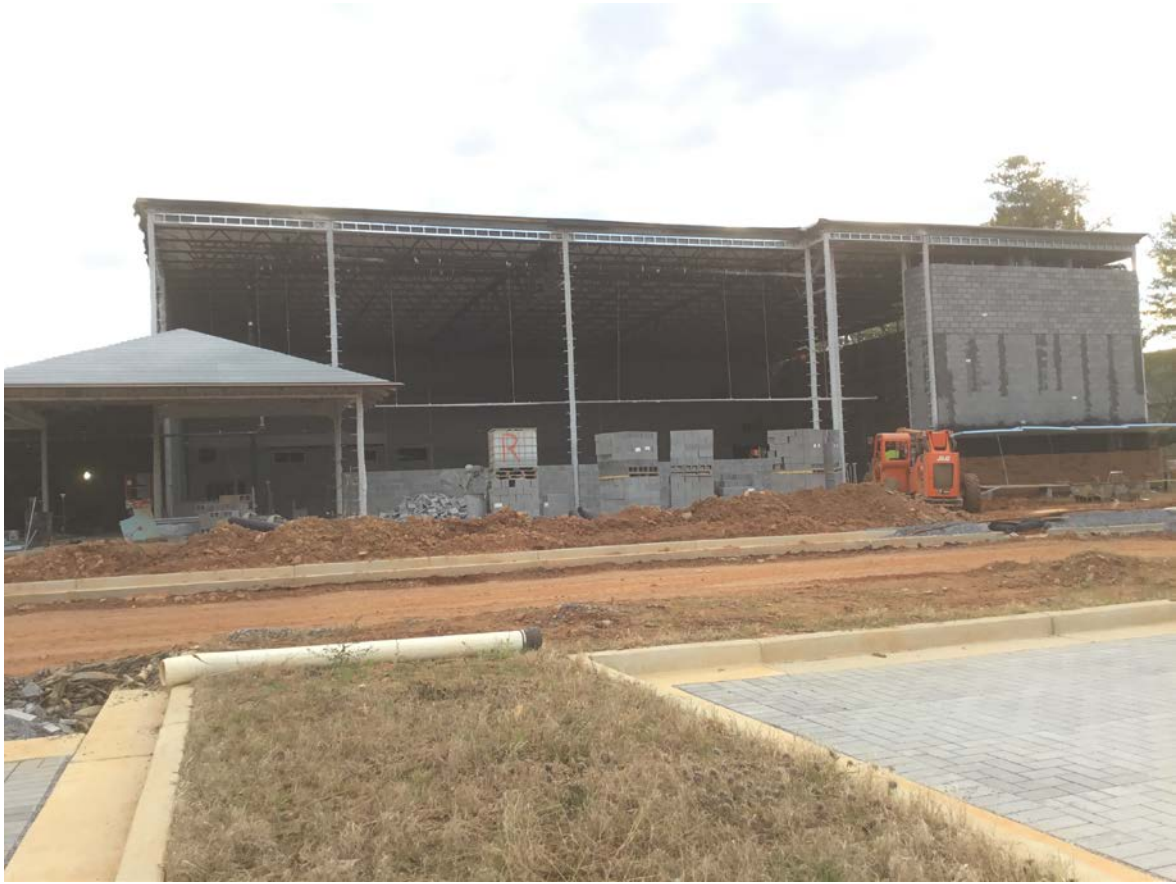
West view at auditorium
