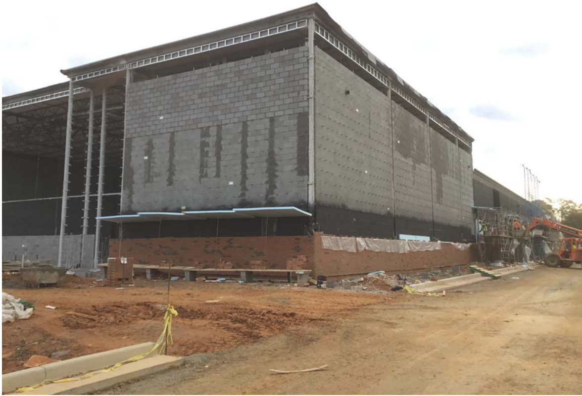
Southwest view at auditorium
