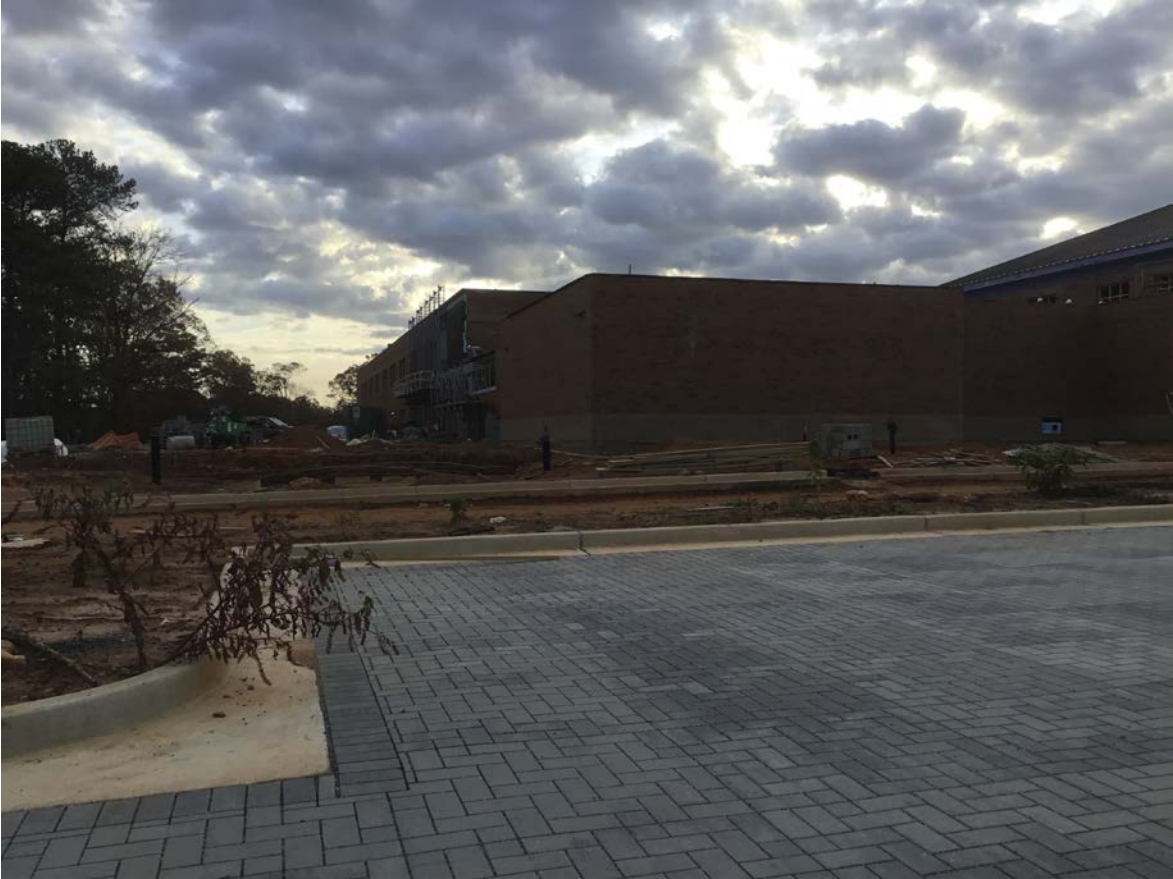
Northwest view at kitchen area
