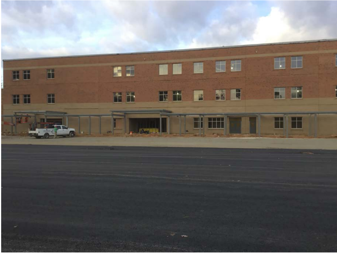
Center view of 3 story
