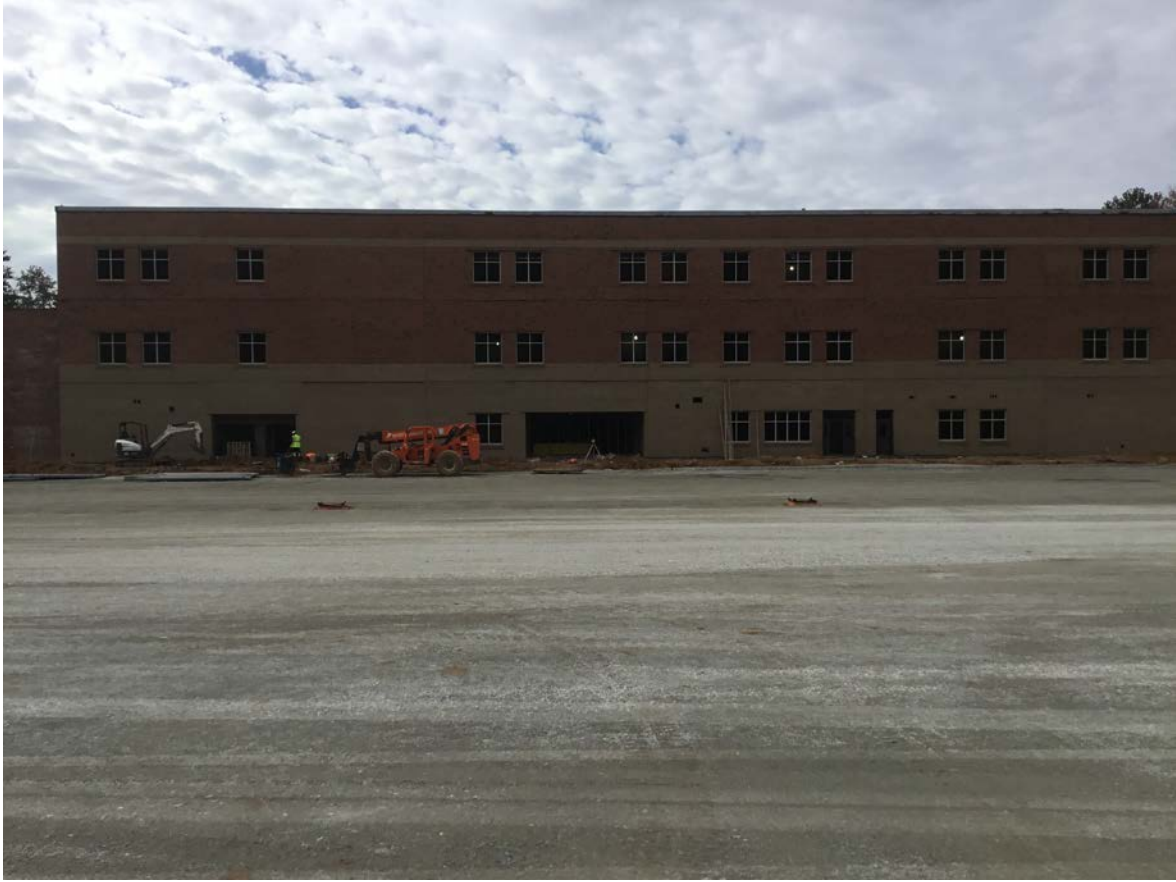
East view of 3 story.
