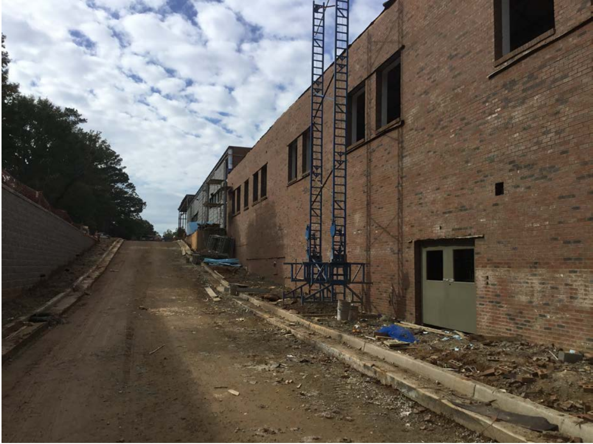
South view of 2 story.
